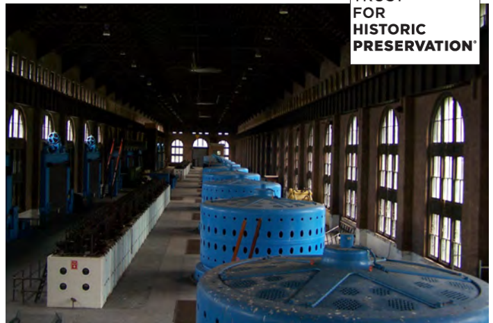
Photo from a tour stop at the historic Canadian Niagara Power plant which is located approximately 50 yards from the Horseshoe Falls.
