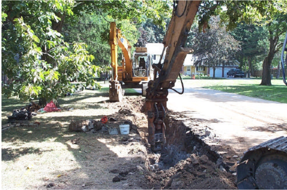
Breaking rock on Sturbridge Lane
