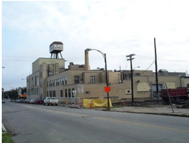
Photos of the project during construction
